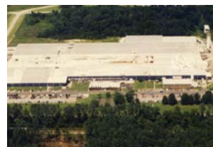
Thrace LINQ (Charleston, South Carolina, USA)
